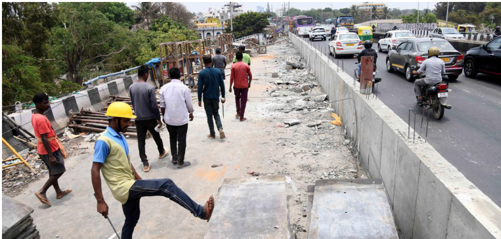
Bangalore Development Authority started the construction work at the flyover up-ramp at Hebbal in Bengaluru on Wednesday. The first day of the diversion witnessed traffic bottlenecks in the area. Only two wheelers will be allowed in the flyover up-ramp
